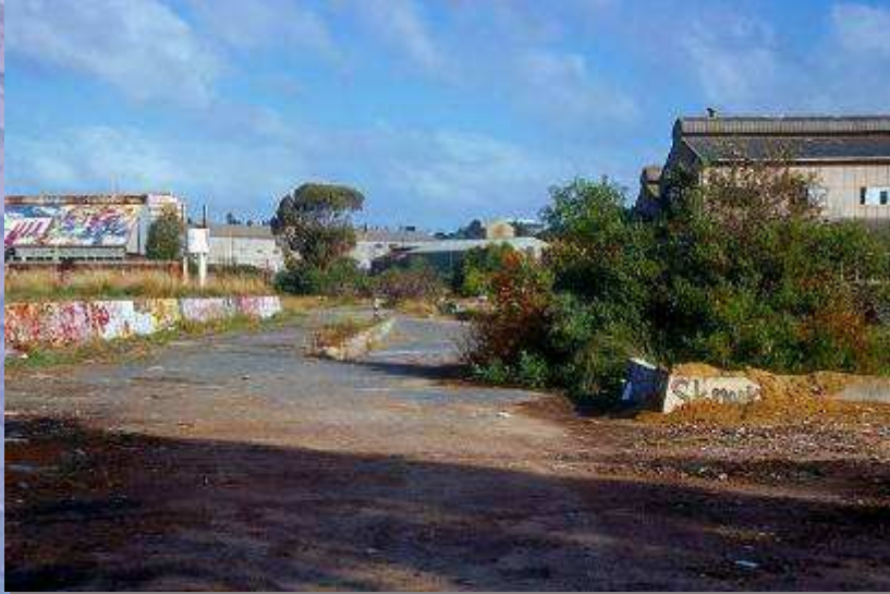
Derelict concrete pipe factory
