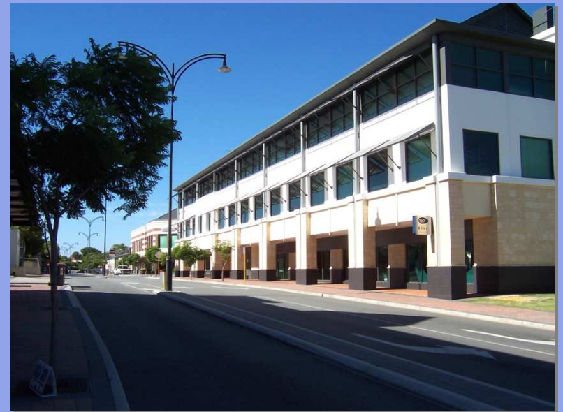
Station Street - Mixed Use Retail/Commercial
