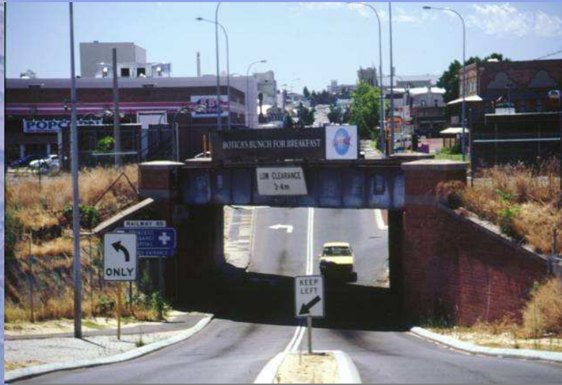
Hay Street Underpass
