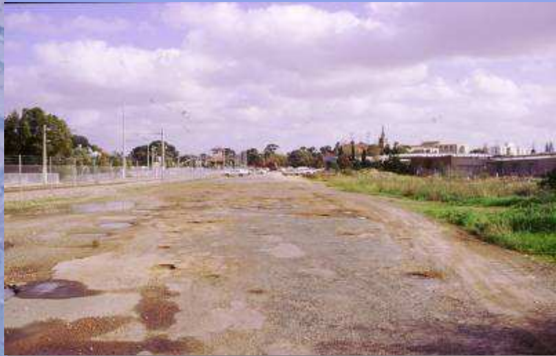
Market Square Parking Area
