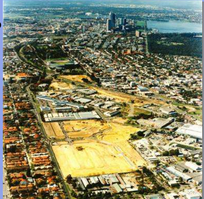
Project area 1996 looking towards city
