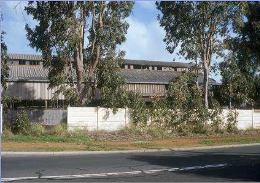
Salvado Road Streetscape
